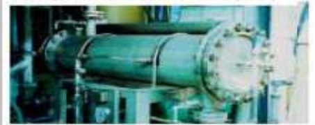
DAF Operation: Separation & Clarification for the factory influent and separating bio-sludge from biological reactor. Courtesy PepsiCo, Frito-Lay International
